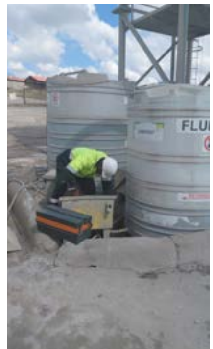
Regular site inspections by Chryso Southern Africa help ensure admixture systems continue to operate reliably, efficiently and at optimum performance.
