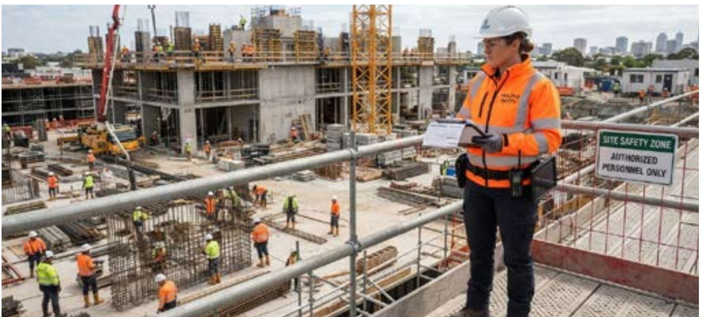
Health and Safety is a main priority and the responsibility of all on site.
