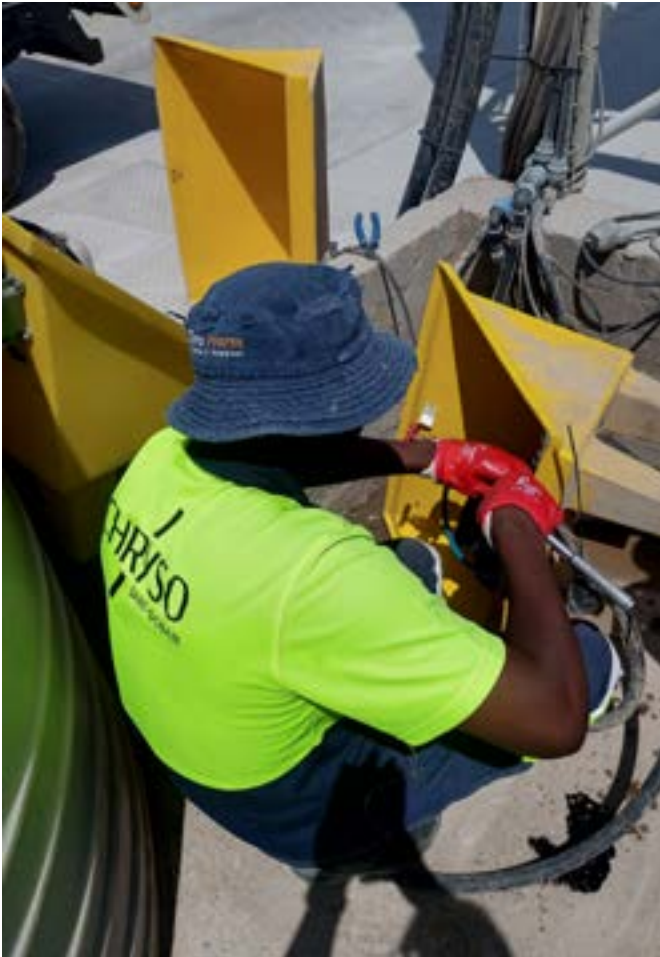
Fast practical on-site support from Chryso Southern Africa helps minimise disruption, reduce downtime and maintain production continuity.
