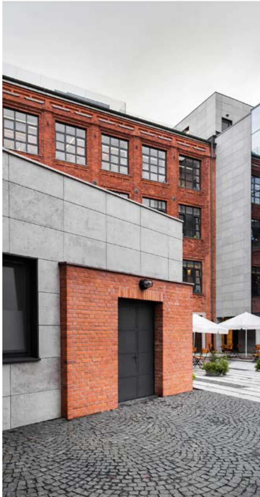
Float cladding achieves its exterior durability through a carefully engineered concrete mix. High-grade cement, pozzolanic binders, fine mineral aggregates and performance-enhancing admixtures combine to form a dense, low-porosity matrix that resists moisture ingress, weathering and prolonged environmental exposure.
