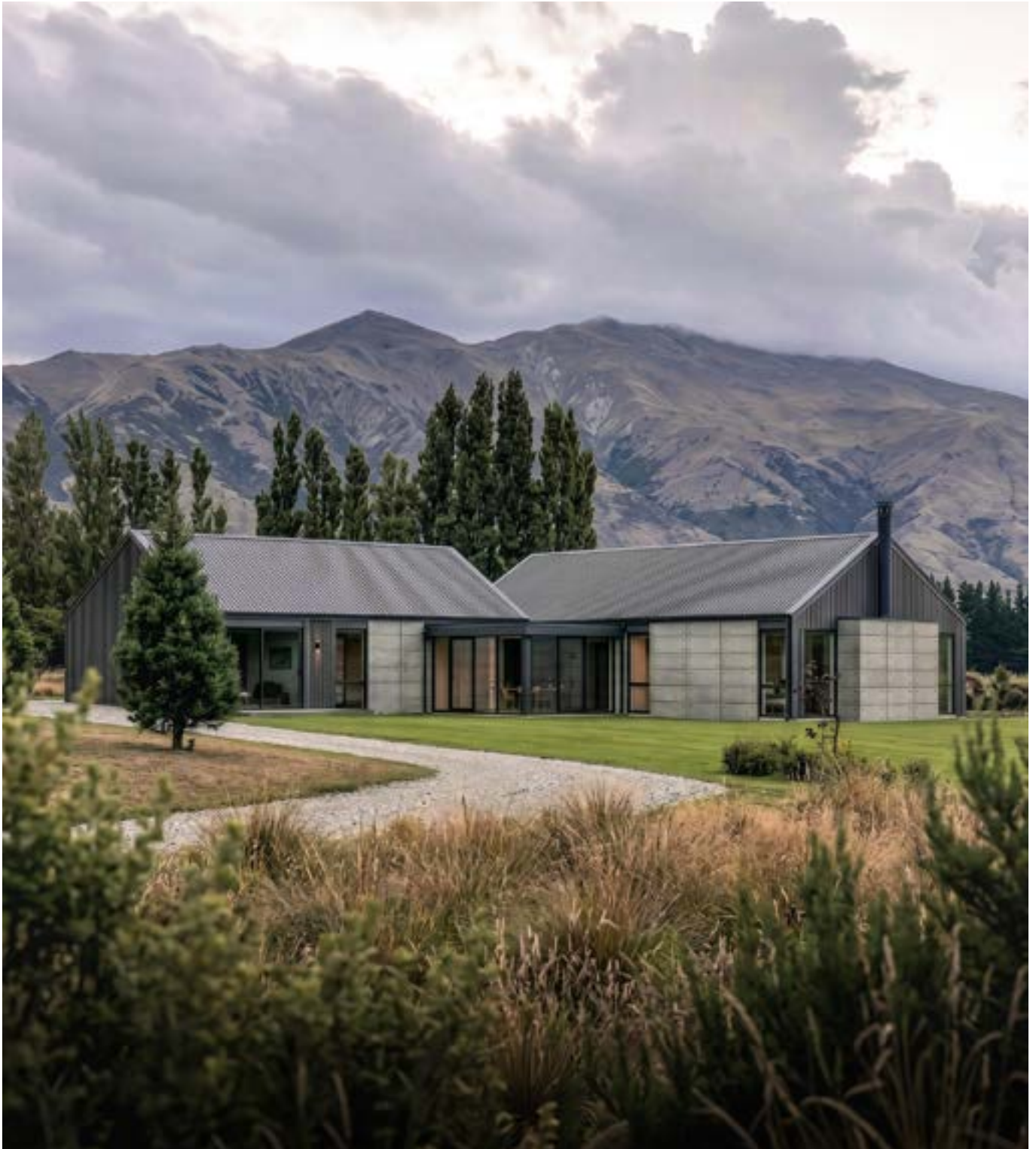
Set against open vegetation and the dramatic Winelands landscape, this residence balances its setting with long-term performance. Float concrete panels create a durable, inherently non-combustible exterior skin, combining the visual depth of cast concrete with lasting weather resistance and material-level fire safety
