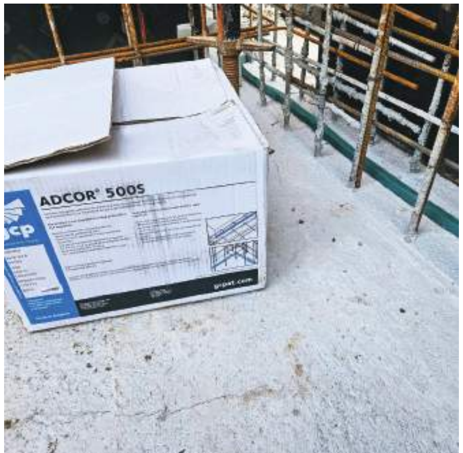
Designed to seal vulnerable construction joints, it helps prevent water ingress where structures are most at risk.
