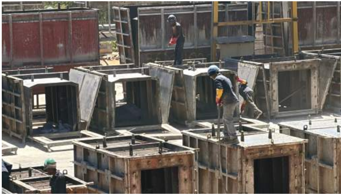
Moulds at Global Precast's yard in Pretoria
