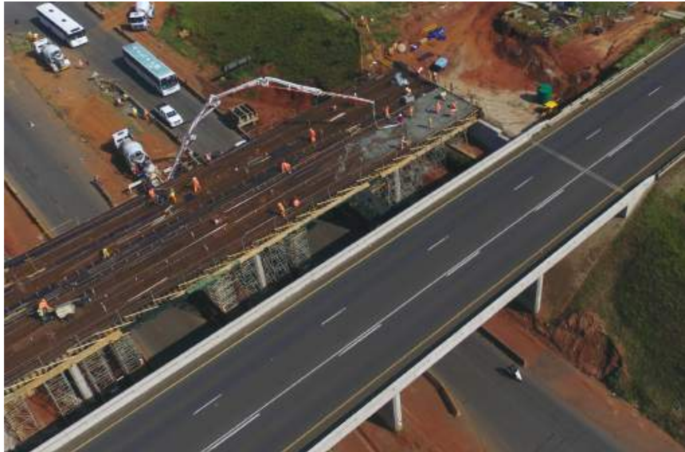
Collaboration across the civil engineering value chain supports fair, transparent and lawful employment practices on construction projects.
