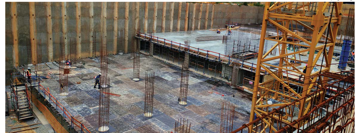
Concor has commenced construction of the 211 Oxford Road development in Rosebank, a fast track future-ready commercial building within the Oxford Parks Precinct, with basement formwork, reinforcement and concrete works progressing.
