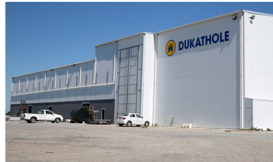
The Dukathole factory, housing the PMSA Ultra 3000 machine, operates on a 24 hours / 6 days per week basis.
