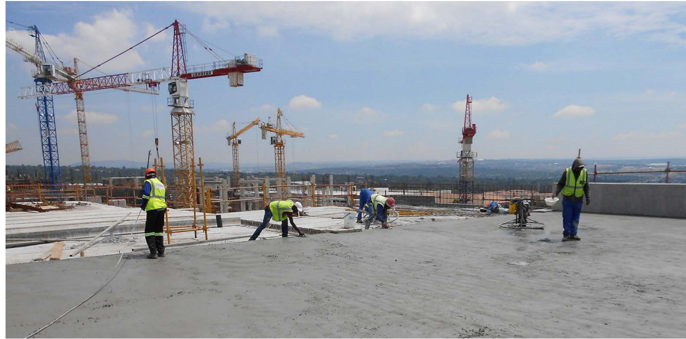
Colloidal silica used to construct durable floor slabs for Teraco's new call centre.
