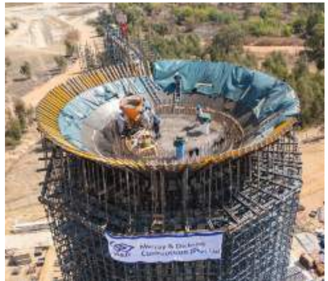
The concrete shaft, 8 metres high and 500 millimetres thick, transitions into a cone-shaped reservoir with a floor up to 1.2 metres thick and a final diameter exceeding 26 metres.
