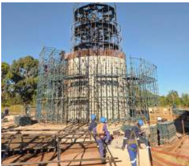
The design of the tower's first 8 metres was particularly crucial, as this section would experience the greatest stress during a seismic event.
