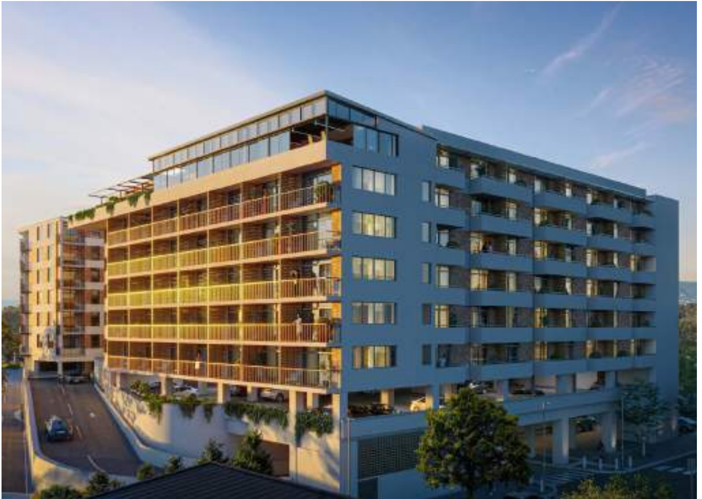
Designed to be 20 to 25% lighter than conventional structures, The Signal reflects Concor's innovative and sustainable construction approach.
