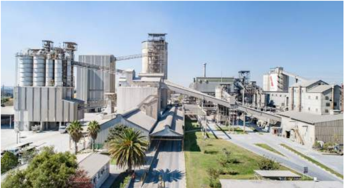
AfriSam continues to prioritise quality across its cement, aggregate and readymix concrete operations.
