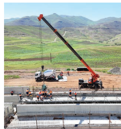
Readymix concrete being poured for manufacture of the precast beams; each beam measures 2,130 m in height and 30 m in length.
