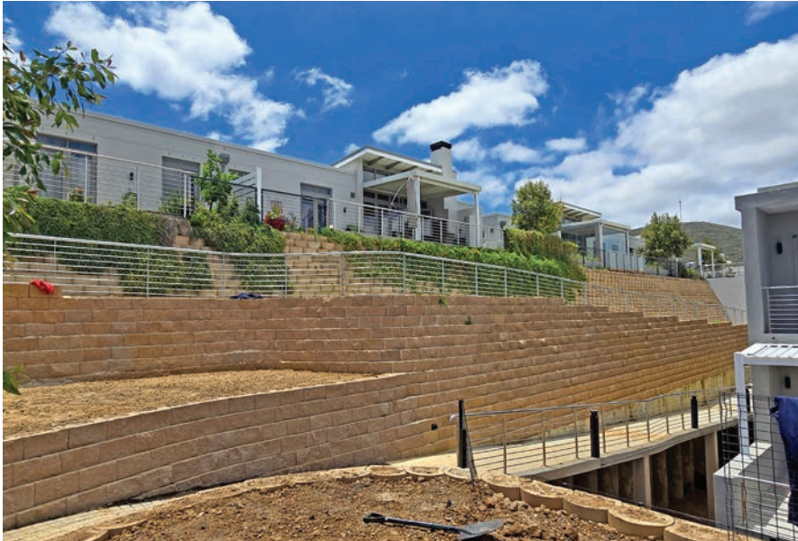
Some of the retaining walls built with Terraforce L-12 Rock Face blocks.
