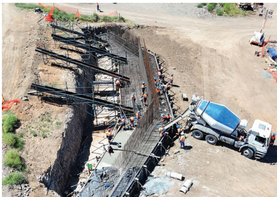
A view of the Khubela Bridge showing the abutment 1 pile cap.
