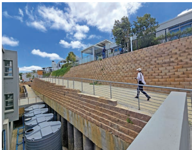
Built on a piled concrete beam, this L-12 Rock Face wall supports a wheelchair path
