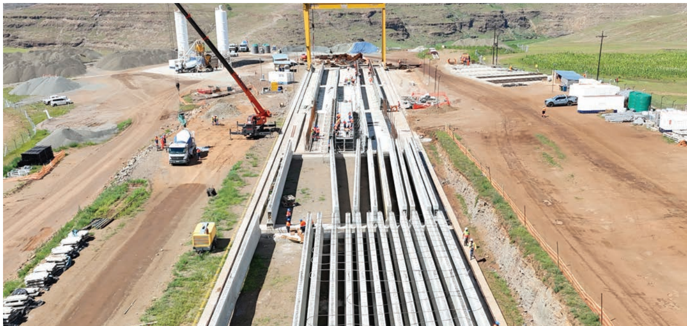
Precast beams are being manufactured on site close to the project's concrete batching plant, allowing the beams to be transported just 1 to 2 km to the bridges.
