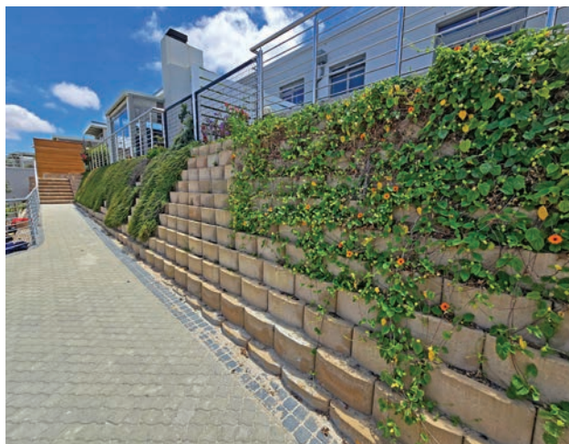
A planted wall built with Decorwall blocks.
