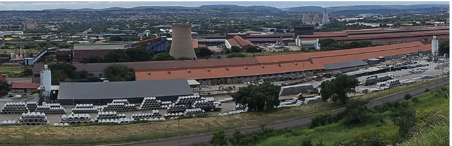
Global Precast's massive site in Pretoria
