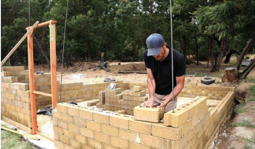
A small house under construction using Click Brick™ blocks.
