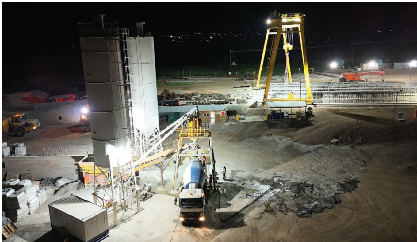
The readymix concrete batch plant during casting of the abutment 1 pile cap for the Khubela Bridge.
