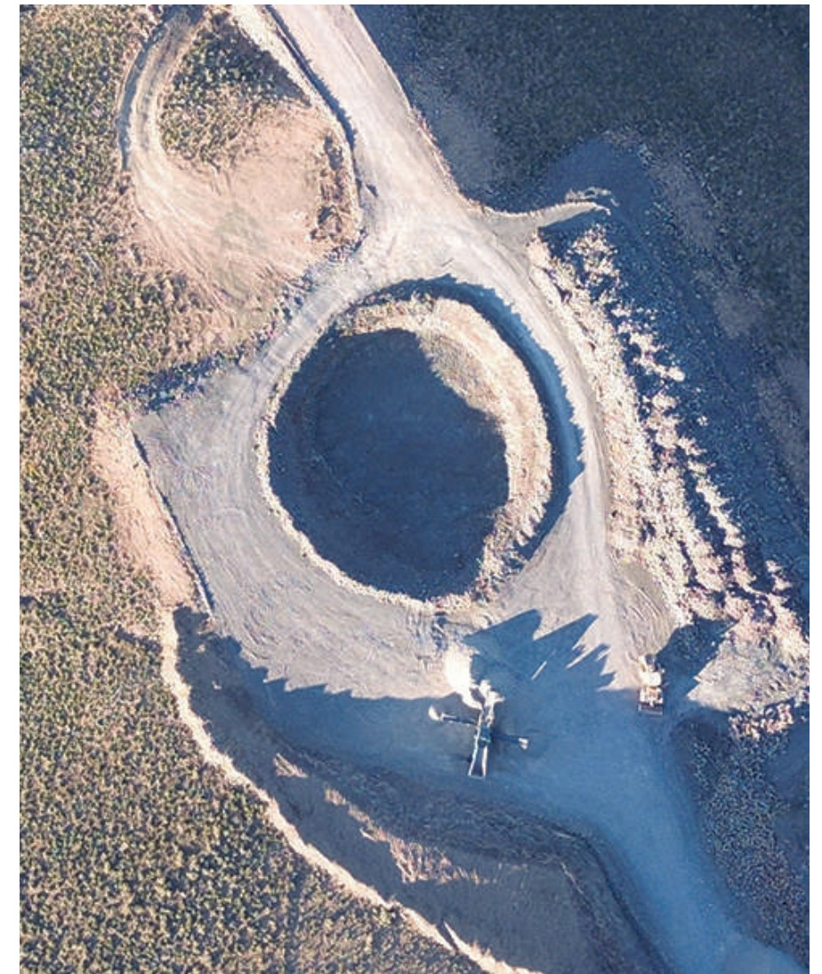
A close-up view captures the excavation of a wind turbine base underway at Karreebosch Wind Farm, where Concor is preparing the foundation to exact specifications based on detailed geotechnical investigations.
