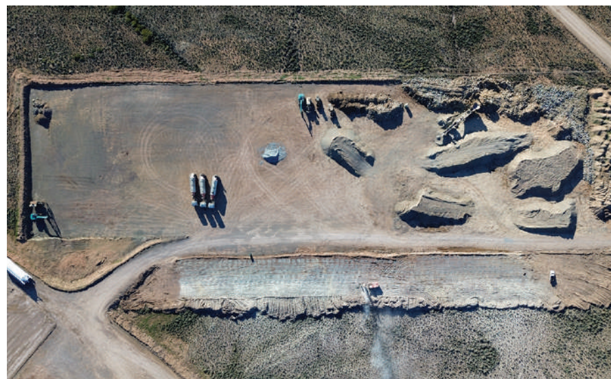
Active crushing operations on the temporary staging area while a drill rig works on extending the platform at the lower end of the site, preparing the area for further construction at Karreebosch Wind Farm.
