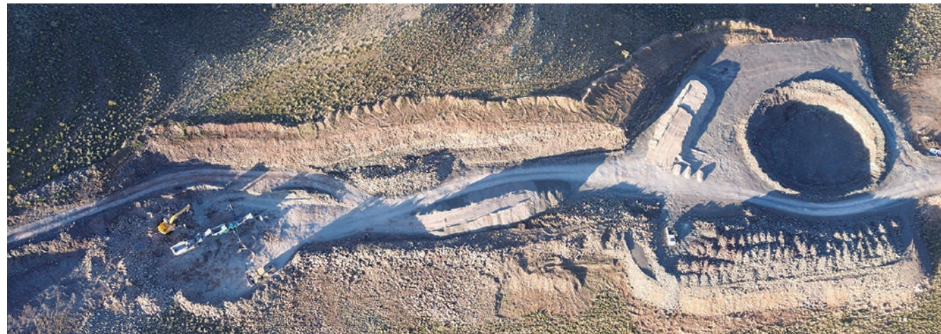
An aerial view captures on-site crushing in operation near one of the wind turbine base excavations at Karreebosch Wind Farm.
