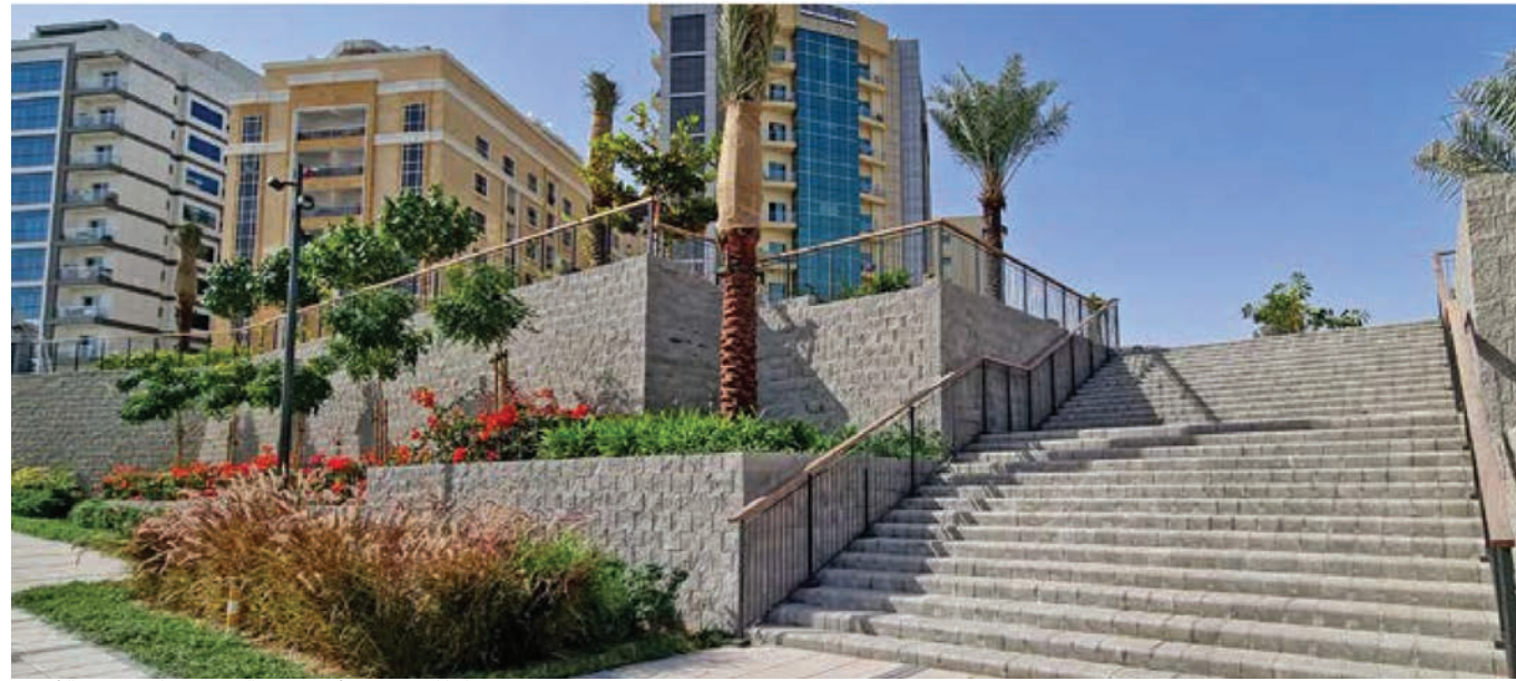
Beautifully constructed retaining walls using Terraforce retaining blocks
