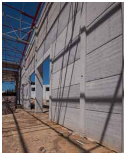
The partially complete southern elevation hollow-core wall.
