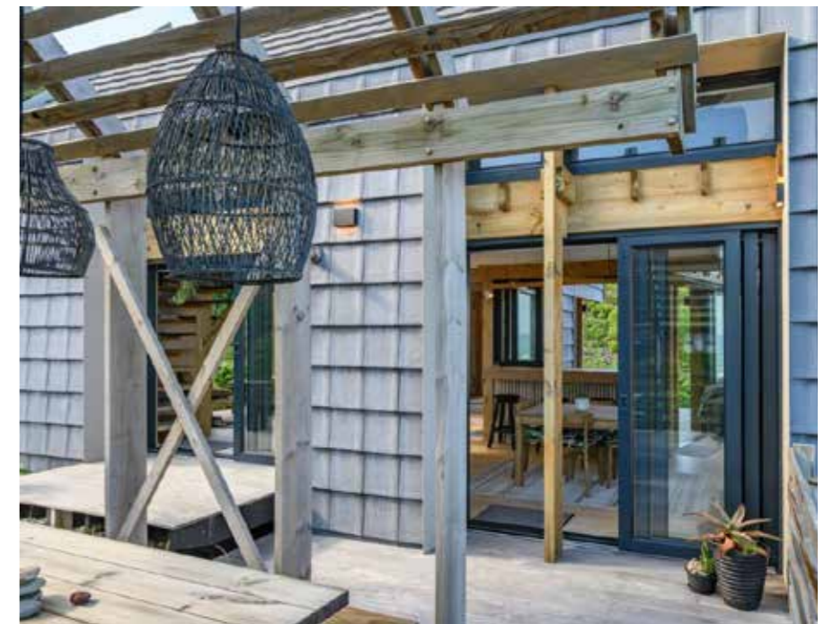
This Beautiful Fantastic was built with Eagle Roof Tiles Slate-grey Shingle roof tiles which were used to clad the wall facades as well as the roof.
