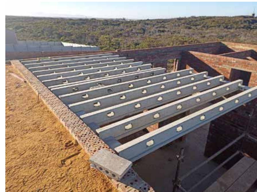
Left: Correctly spaced T-beams. Above: Filler blocks installed.
