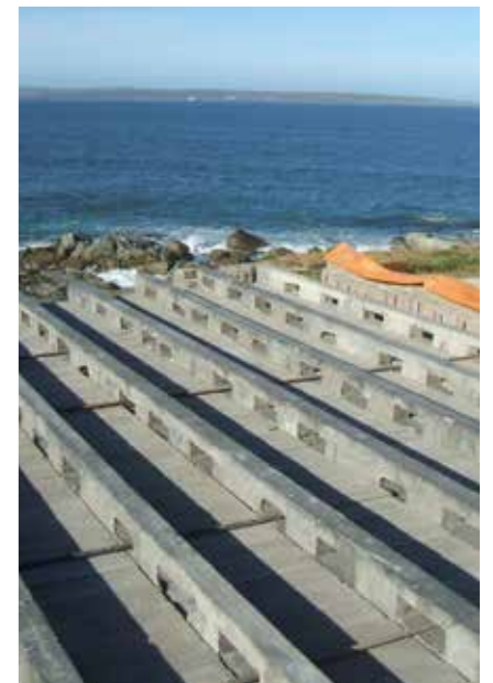
Left: Correctly spaced T-beams. Above: Filler blocks installed.
