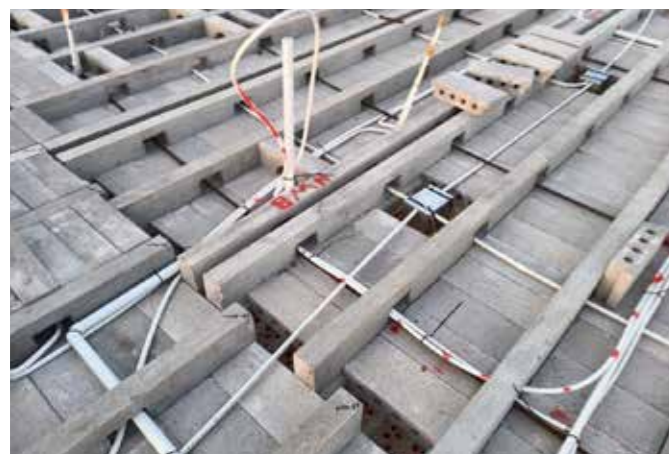
Top: A lateral view of a completed DRIDEK floor. | Left: Completed services and cross-beam rebar. | Right: Compression blocks in place providing cavities for cross-beam casting.
