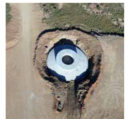
Main Image: Each turbine base constructed measures over 20 m in diameter and is around 3,3 m deep. More complex in design and execution, the hollow foundation allows for the inclusion of ducts and facilitates the post-tensioning of cables for the concrete tower. The construction of hollow foundations is more labour intensive and requires more formwork and steel reinforcing. Top: Each of the San Kraal wind turbine base foundations used a total of 64 tons of reinforcing steel and required over 400 m 3 of 45 MPa concrete – with an additional 18 m 3 of 50 MPa concrete in the plinth. Above: Concor recently completed the final foundation cast for the San Kraal Wind Energy Facility in Noupoort, as part of the Koruson 1 Cluster.
