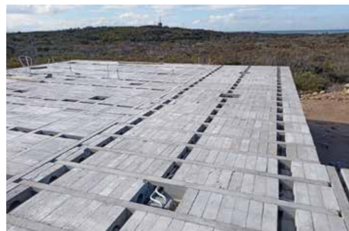
Top: A lateral view of a completed DRIDEK floor. | Left: Completed services and cross-beam rebar. | Right: Compression blocks in place providing cavities for cross-beam casting.
