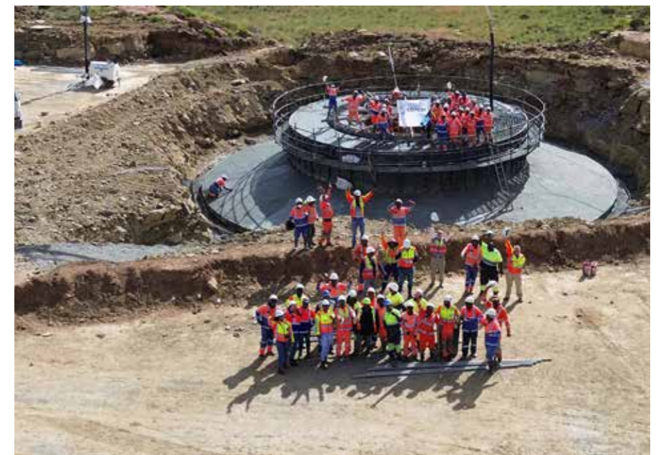
Main Image: Each turbine base constructed measures over 20 m in diameter and is around 3,3 m deep. More complex in design and execution, the hollow foundation allows for the inclusion of ducts and facilitates the post-tensioning of cables for the concrete tower. The construction of hollow foundations is more labour intensive and requires more formwork and steel reinforcing. Top: Each of the San Kraal wind turbine base foundations used a total of 64 tons of reinforcing steel and required over 400 m 3 of 45 MPa concrete – with an additional 18 m 3 of 50 MPa concrete in the plinth. Above: Concor recently completed the final foundation cast for the San Kraal Wind Energy Facility in Noupoort, as part of the Koruson 1 Cluster.
