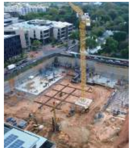
MAIN IMAGE: Concor is constructing two office buildings integrated with basement parking and a retail development on the ground floor in the Oxford Parks Precinct. ABOVE: Raft foundation work is underway for the Oxford Parks Block 2A Phase I project.
